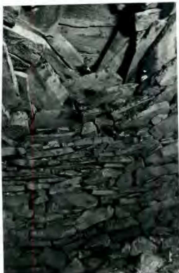
Plate 14. Interior of a corbelled hut showing roof construction. Sedan, Lindley District.
