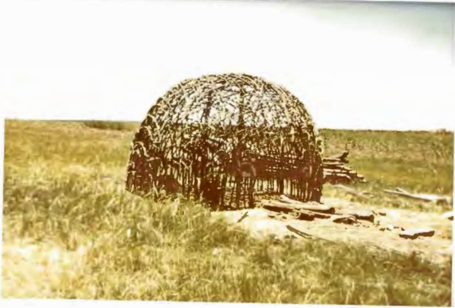
PHOTO 4 ROOF FRAMEWORK
