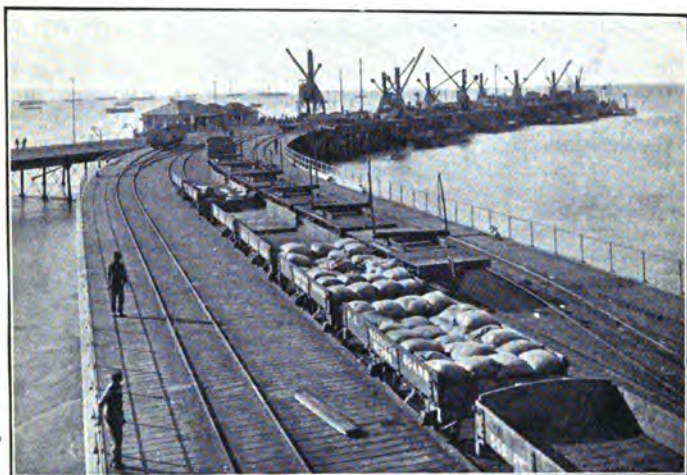
NORTH JETTY, PORT ELIZABETH.
