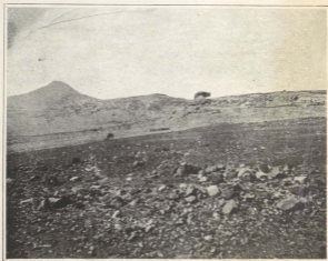
Kueneig from the west, Balokoa ruins in foreground.
