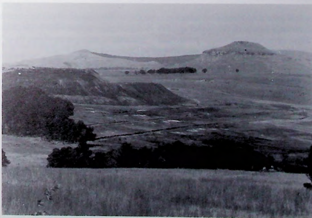
Plate 8: A view of the anthracite washing plant at the head of iShoba vlei. Note the slime dams and cut-off drains that have been constructed in an effort to contain run-off from the dumps.
