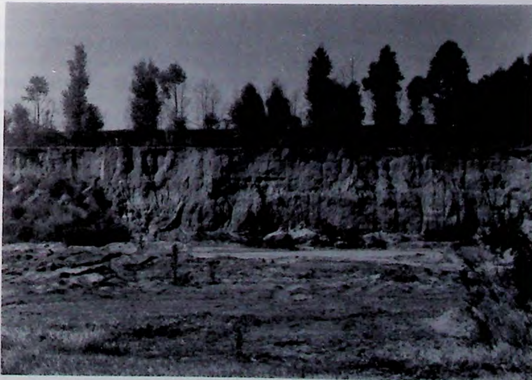
Plate 24: Bank erosion of the Sandspruit River in quaternary sub-catchment No. W214 has probably been exacerbated by wetland destruction upstream.
