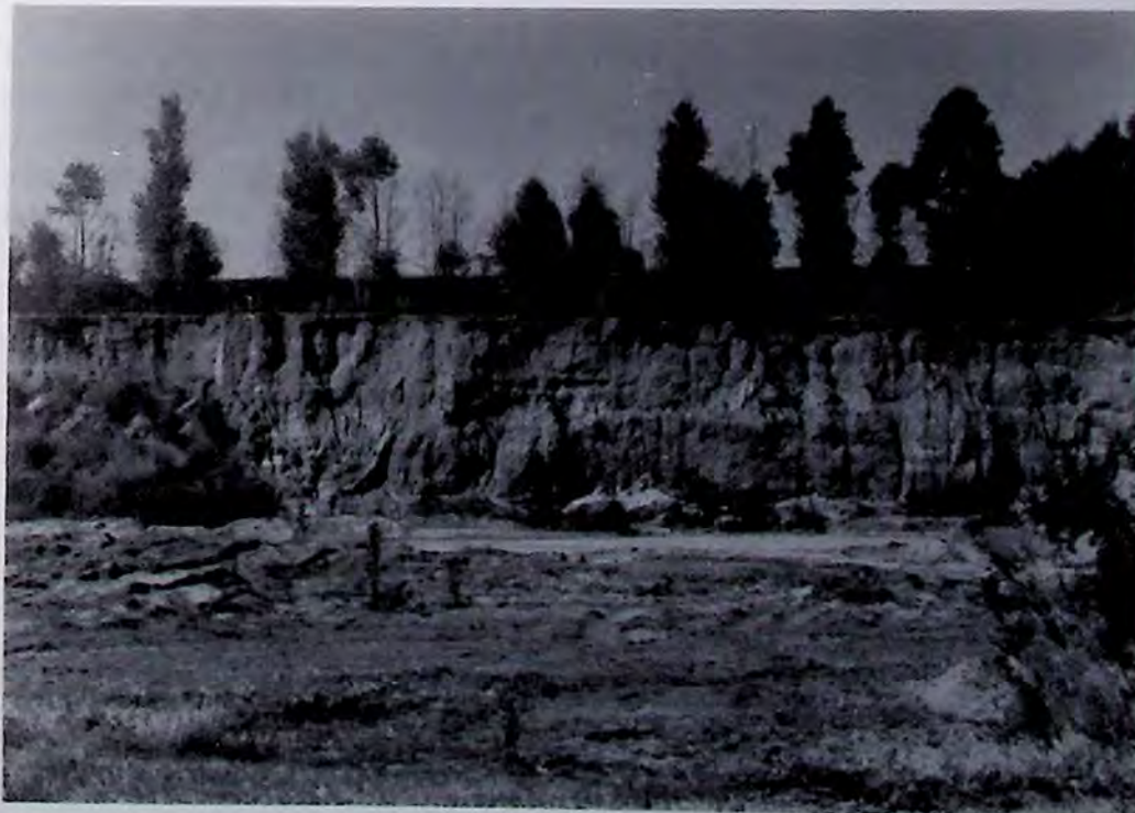
Plate 24: Bank erosion of the Sandspruit River in quaternary sub-catchment No. W214 has probably been exacerbated by wetland destruction upstream.
