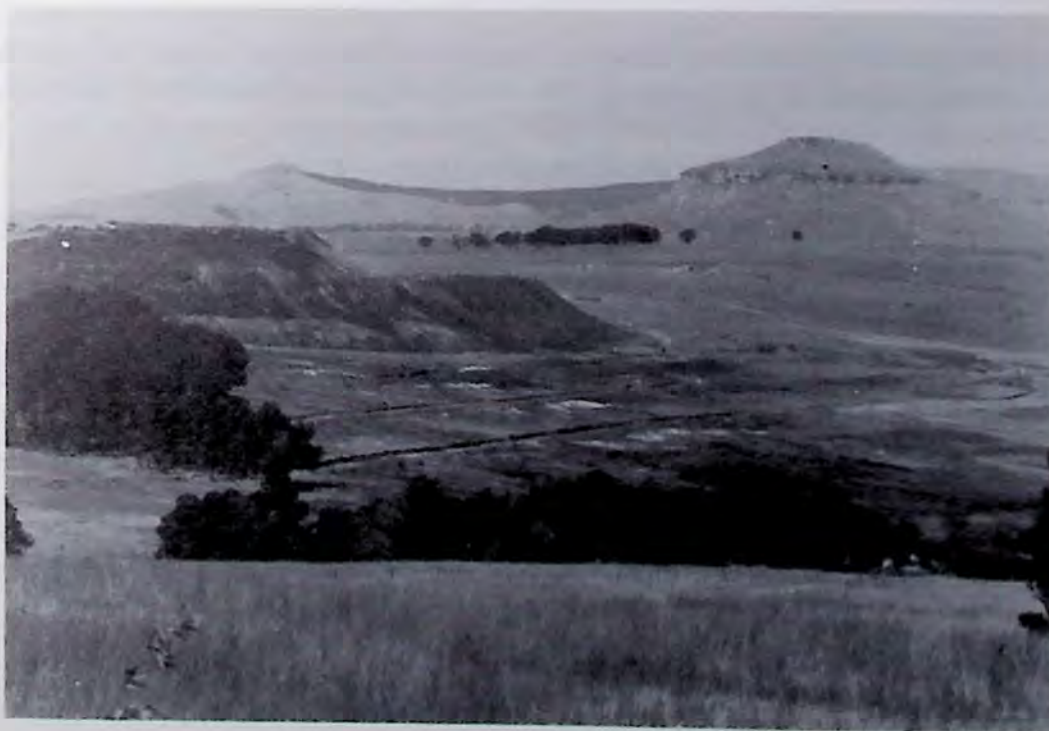
Plate 8: A view of the anthracite washing plant at the head of iShoba vlei. Note the slime dams and cut-off drains that have been constructed in an effort to contain run-off from the dumps.
